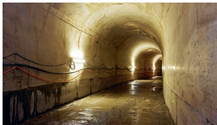
A bypass tunnel near Tiefencastel transports the sediment downstream in the event of a flood. (Photo: ewz-Medienarchiv/Matthias Kunfermann)
