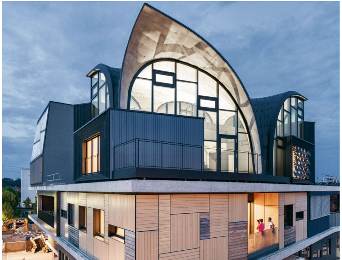
The HiLo unit with its doubly curved concrete roof and the adaptive façade with solar cells on the NEST. > Empa
